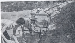
Braving the scorching heat, campers pitch into work. They are digging a drainage system for the pasture.
